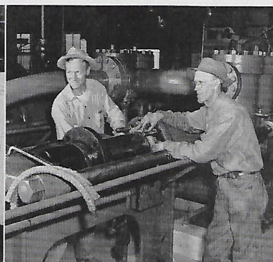
(L-R) Ray Dooley makes his hourly report to the dispatcher. Arthur Dean and Earl Calder equip a pump with new packing. George Faustino gauges a 1¼-million barrel ground-storage reservoir.
