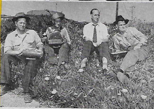
Top to bottom: Nick T. Ugrin, who by coincidence has just been named superintendent of Northern Division Pipe Lines, is the author of this pipe line narrative. Glenn Wood and Peter Glynn connect a new receiving line at Rio Bravo Pump Station. Out for lunch at Avila are (L-R) H. R. Martinson, John C. Calhoun, William Mercer and William Esplin, whose service records run 15, 30, 31 and 38 years respectively.
