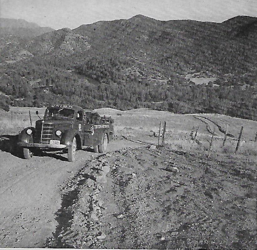
Enroute with a full load of fuel and lubricants to the new highway now under construction, a Company truck pauses above a portion of Kings River Valley soon to be flooded by the new Pine Flat Dam.
